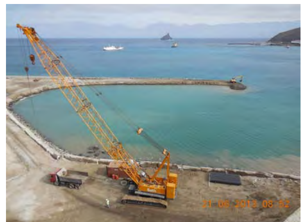
General view of the port area with embankment construction in progress
