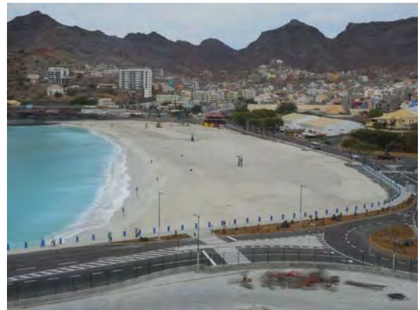
Laginha Beach after completion of sand filling
