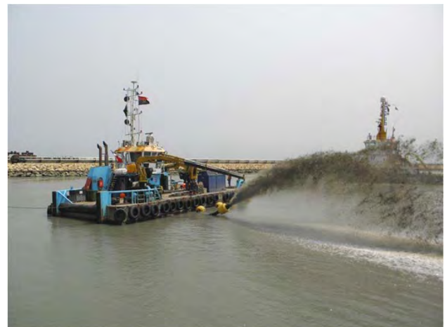
Dredging with DOP pump
