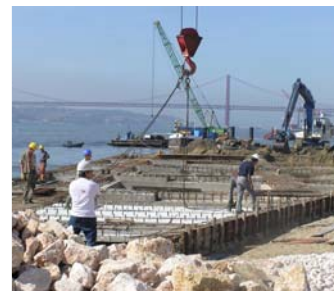
Vista geral das estacas de guiamento. General view of piling to guide floating pontoons for the Cais do Sodré Interface in Lisbon.
