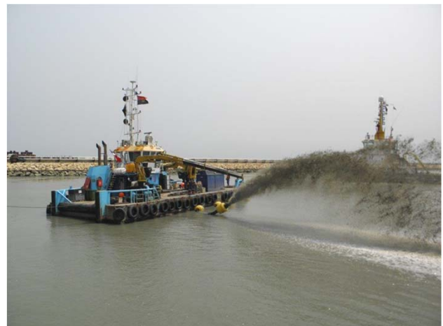
Dredging with DOP pump
