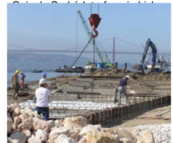
Vista geral das estacas de guiamento. General view of piling to guide floating pontoons
