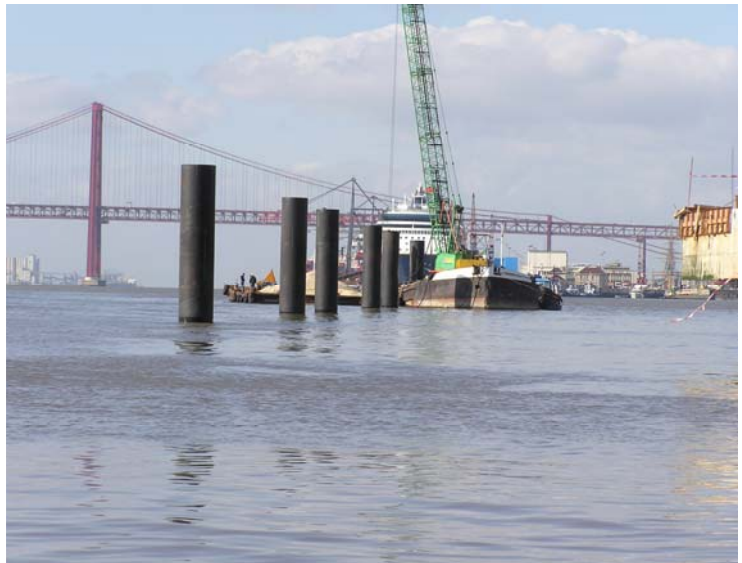
Vista geral das estacas de guiamento. General view of piling to guide floating pontoons
