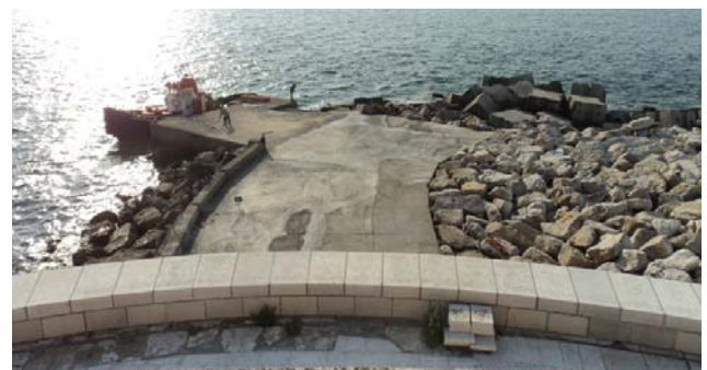
View of the works (Photo by Manuel Garcia)
