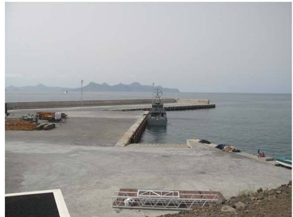
Zone of berths after completion of the work
