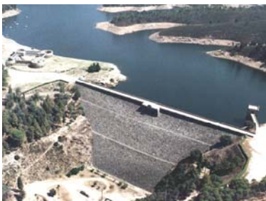
Pego do Altar Dam Built by SETH in 1949
