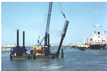
Petrogal - Aveiro Marine pile driving
