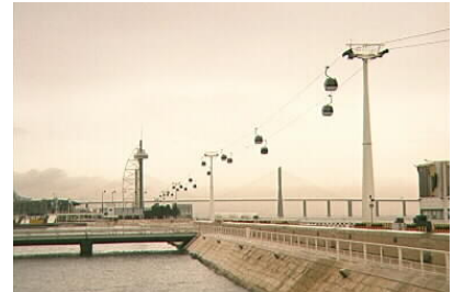
EXPO '98 Aerial Ropeway
