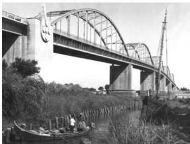
Marechal Carmona Bridge Built by SETH in 1951
