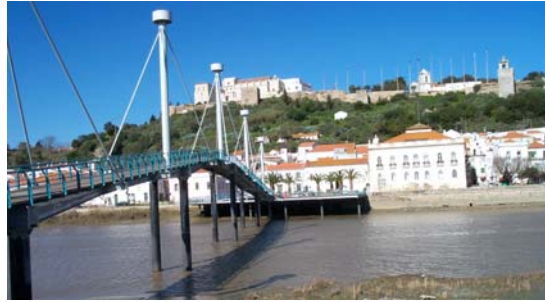
Pedestrian Bridge, Alcácer do Sal, Portugal Pylons: tubular driven piles (Ø 708 and 508 mm)
