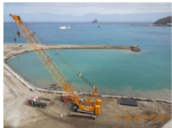
General view of the port area after intervention of this work
