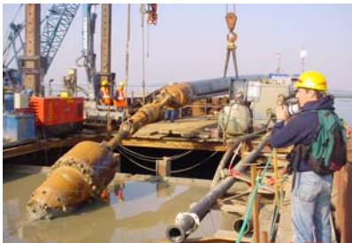
Sines-Setúbal Gas Pipeline HDD Works at Sado River Crossing Pull-Back Operations
