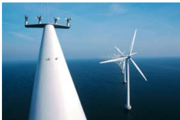
Offshore Wind Turbines Denmark
