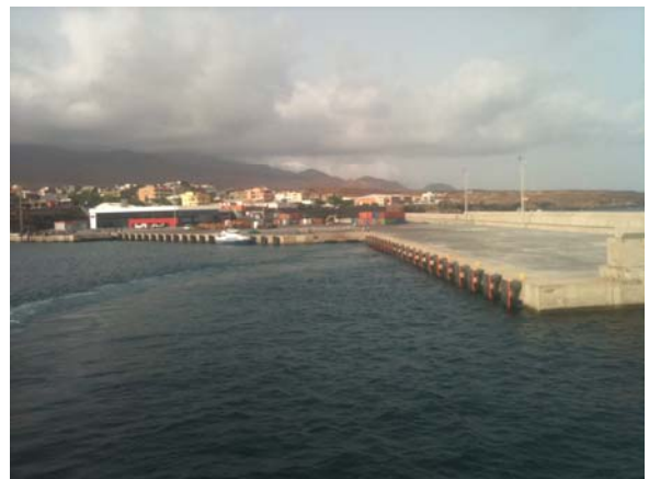
General view of the port area after project conclusion
