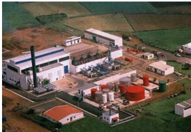
EDA - Diesel Power Plant Addition Belo Jardim, Terceira - Azores
