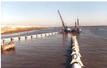
Marine works Water intake, Valorsul
