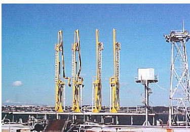
NATO POL Pier Lisbon, Portugal Loading arms replacement
