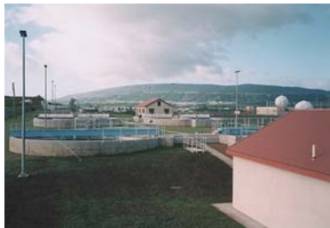
U.S. Navy Lajes Field, Azores Wastewater Treatment Plant
