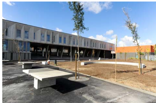
Overview of the school buildings
