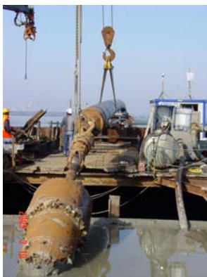
Sines-Setúbal Gas Pipeline HDD Works (Sado River)
