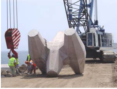
32 T Core-Loc® Praia da Vitória Harbour Breakwater Largest in the world
