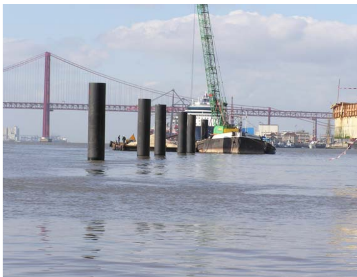
Vista geral das estacas de guiamento. General view of piling to guide floating pontoons for the Cais do Sodré Interface in Lisbon.
