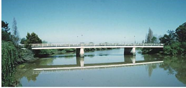
The “Vala Nova” Bridge The first pre-stressed concrete bridge in Portugal Built by SETH in 1954
