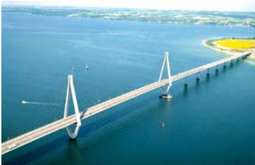
Farøbroen Bridge Denmark
