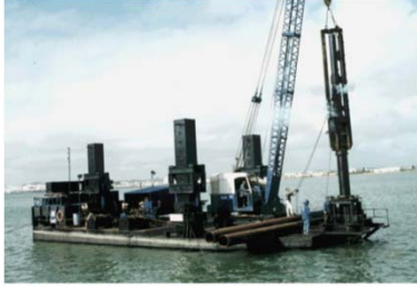
Jack-up platform "Valeira" Marine pile driving
